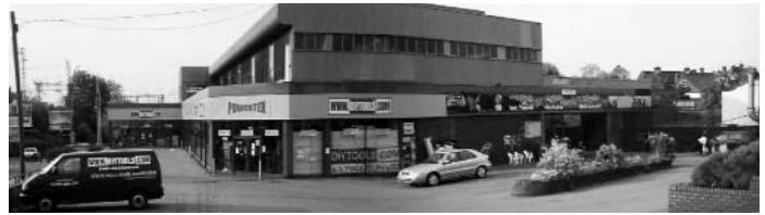
The JR Tagger site is being targetted by developers again.
